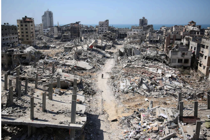
Figure 5: Street with apartment buildings in the Gaza strip, as of July 2025 56
